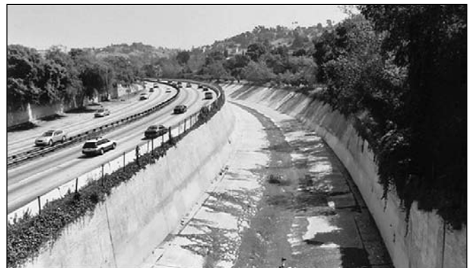
Extreme river-engineering: The Los Angeles River has been reduced to a concrete channel.
