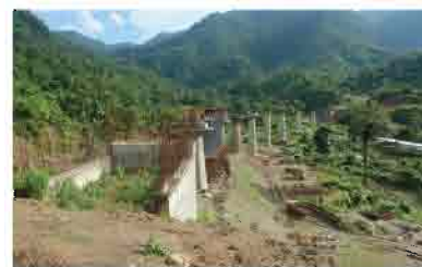
Construction work of a bridge in progress in Lumding-Silchar Section.
