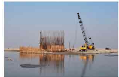
A view of Bogibil Bridge project, Northeast Frontier Railway.
