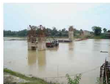
Construction work of a bridge in progress in Lumding-Silchar Section.
