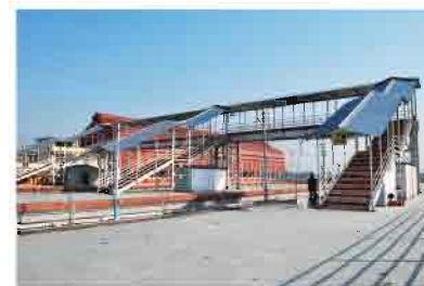
A view of Foot-Over-Bridge at Dibrugarh Station, N.F. Railway.
