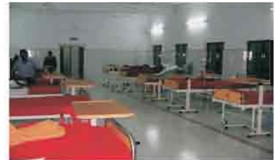
A view of renovated Ward No.2, Central Hospital, Bilaspur, South East Central Railway.
