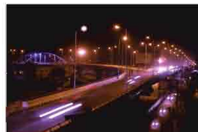
View of a Rail-Over-Bridge in Bihar at LC-75 (Dhanus Setu).
