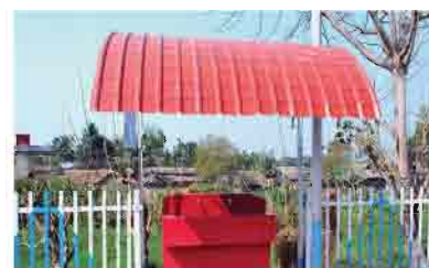
Drinking water facilities at Tinsukia Station, Northeast Frontier Railway.
