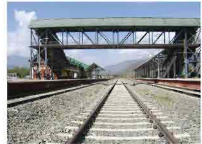
A view of Foot-Over-Bridge of way side Station in Qazigund-Baramula Section.
