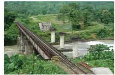
Tunnel & bridge construction work in progress in Lumding-Silchar Section.
