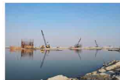
A view of Bogibil bridge project, Northeast Frontier Railway.
