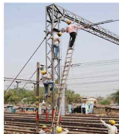
OHE maintenance on North Central Railway.
