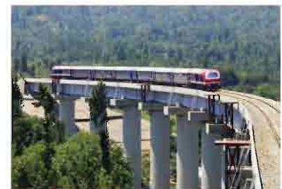
J&K rail link project.
