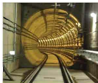
Inside view of a tunnel, DMRC-Delhi.
