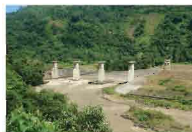
Construction work of a bridge in progress in Lumding-Silchar Section.
