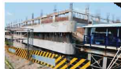
Construction of new station building at Andheri Railway Station, Western Railway.
