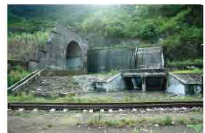
Tunnel & bridge construction work in progress in Lumding-Silchar Section.
