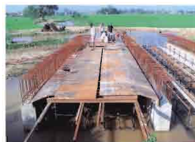
Form work in progress at Bridge No. 575, (DFCCIL).
