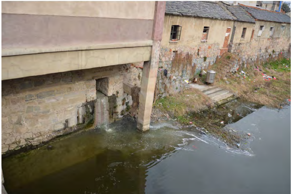
Household wastewater discharge along the bank of Zhegao River, one of the rivers flowing into Chao Lake (Anhui Chao Lake Environmental Rehabilitation Project Management Office)
