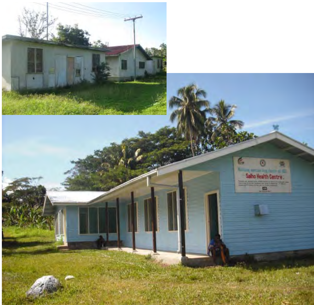
Saiho Health Centre—one of the aid posts renovated by the pilot HIV/AIDS Prevention and Control in Rural Development Enclaves Project, with the old center inset.
