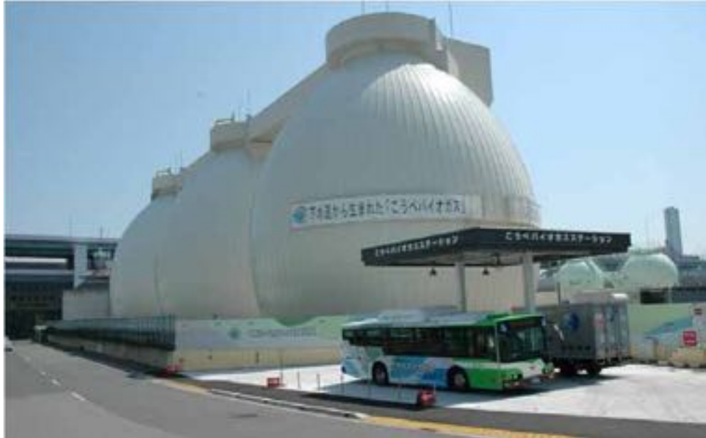
Digestion tanks and Kobe Biogas Eco-station.
