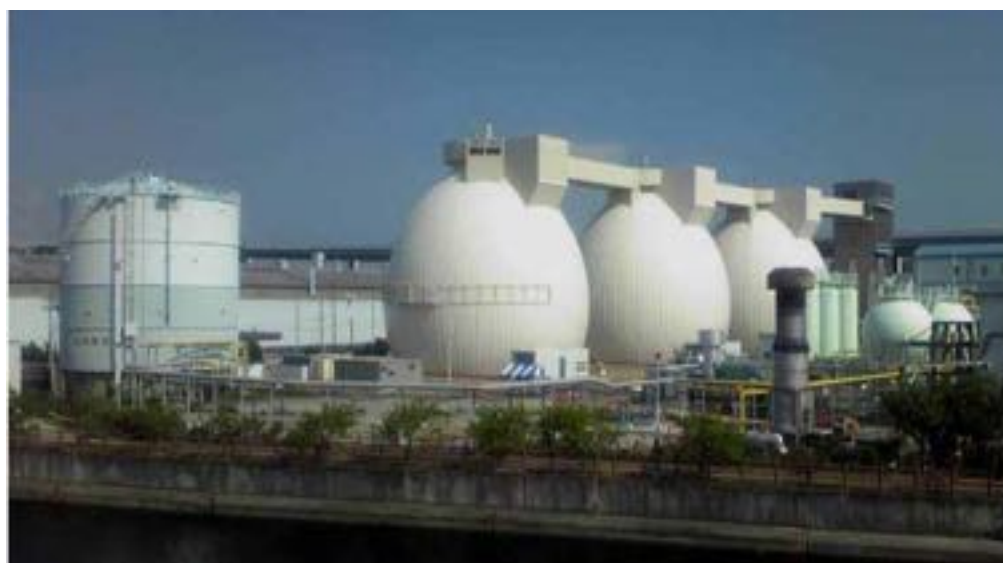
Kobe gas is produced at Higashinada WWTP.
