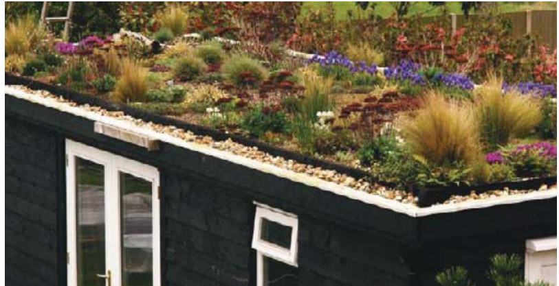
A green roof
