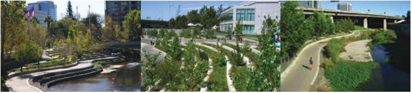
River Bank Terracing and Vegetation as Part of a Green Infrastructure Network in Guadalupe River Park in San Jose, California, United States
