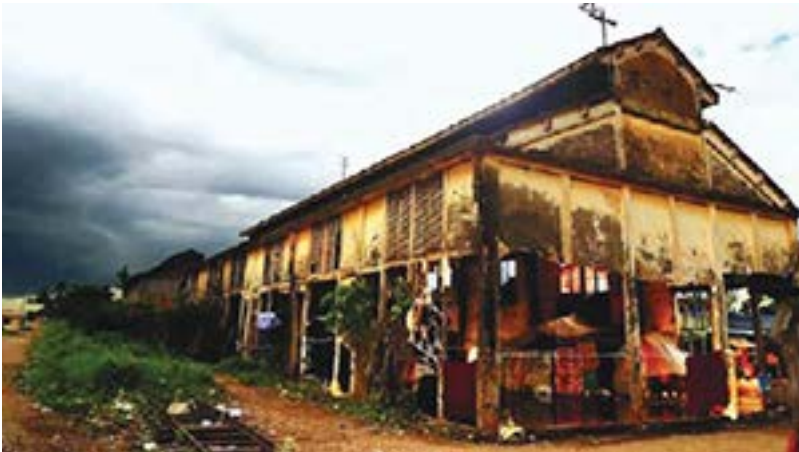
The rail yards and maintenance buildings
