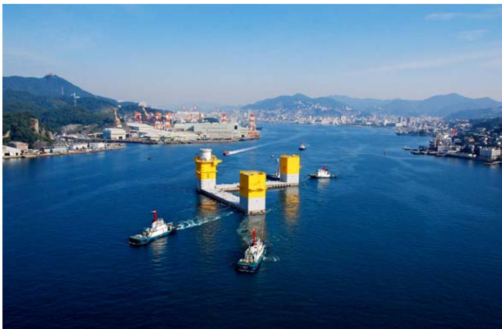
Fukushima 7MW floater in Nagasaki © FukushimaFORWARD MHI
