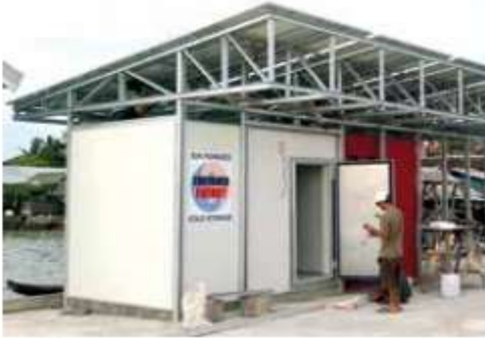
☒ Solar powered cold storage system
