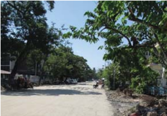
Secondary road outside the city center
