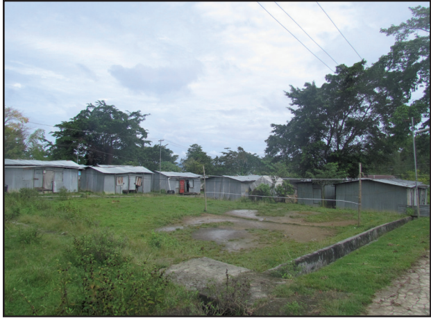
Pic: 2 (Great Nicobar) The post-tsunami Nicobarese intermediate/ temporary shelters at Rajiv Nagar.
