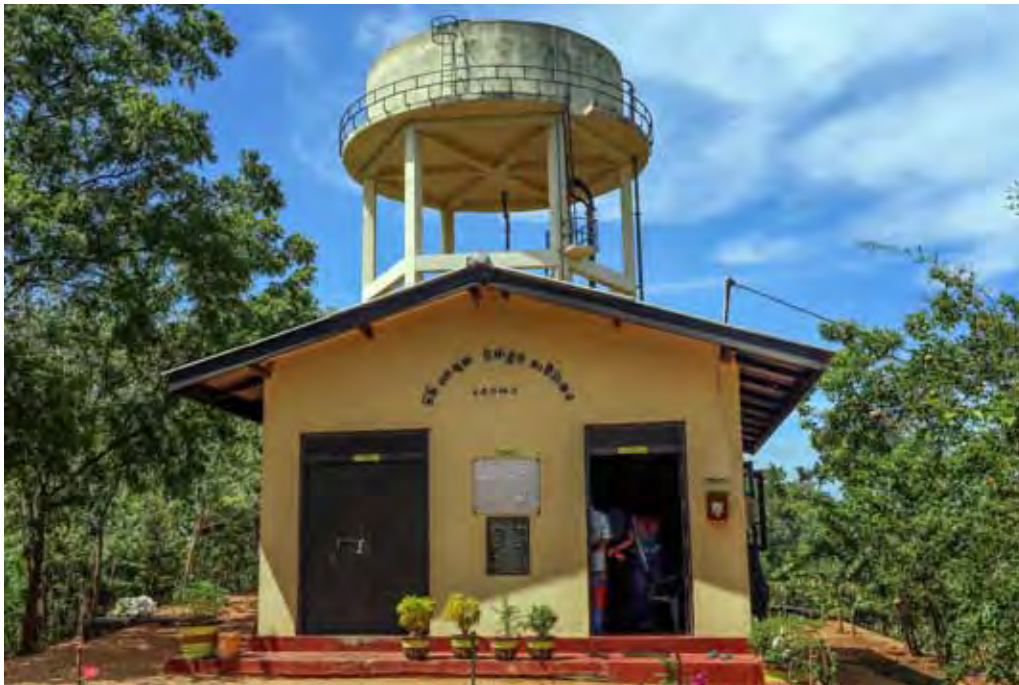
The office building and the water tank of the Polonnaruwa-Ikiriwewa rural water supply system
