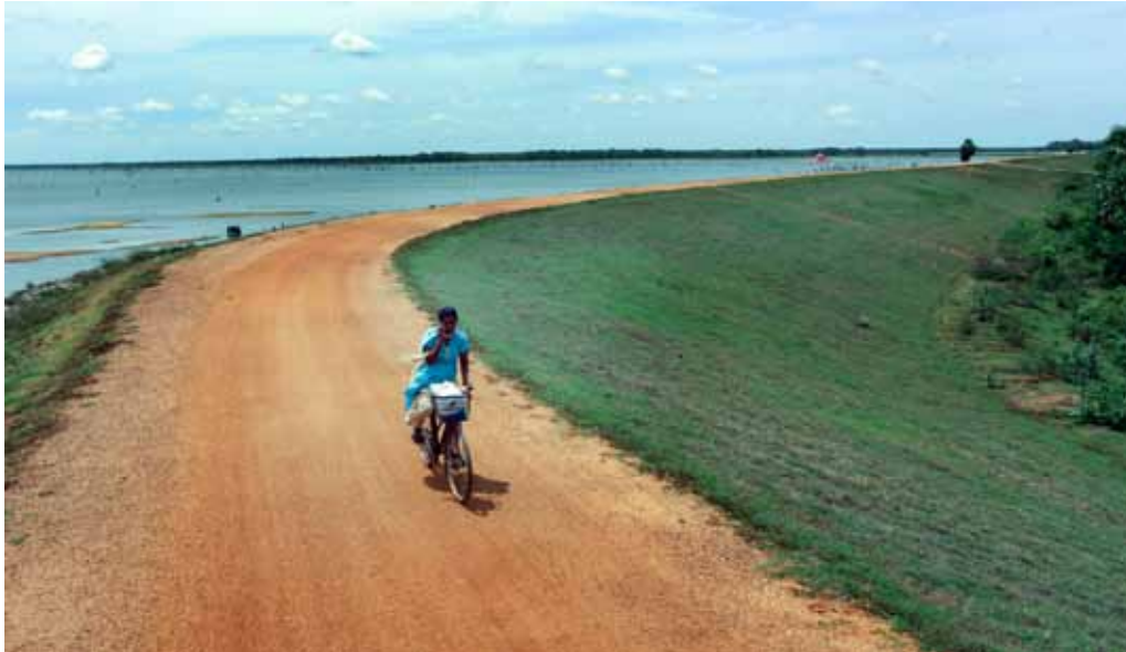
An ADB-supported project improved the Vavunikulam reservoir.
