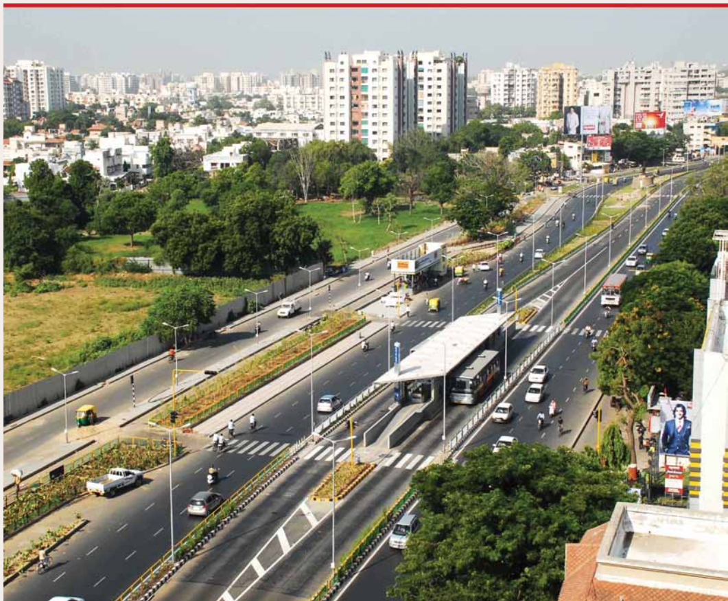
FIGURE B4.4.1 Bird's eye view of the BRTS station at Jhansi ki Rani junction, Ahmedabad, India
