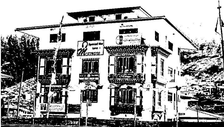
New residential buildings converted into offices and commercial spaces
