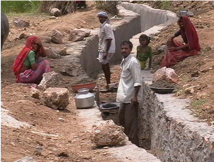
A field channel (Ghaura) constructed in Bhalokaguda GP in Girwa block in Udaipur district
