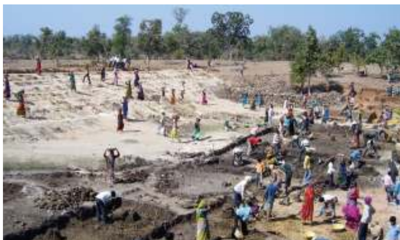
Earthen dam under construction under MGNREGA in Bagli
