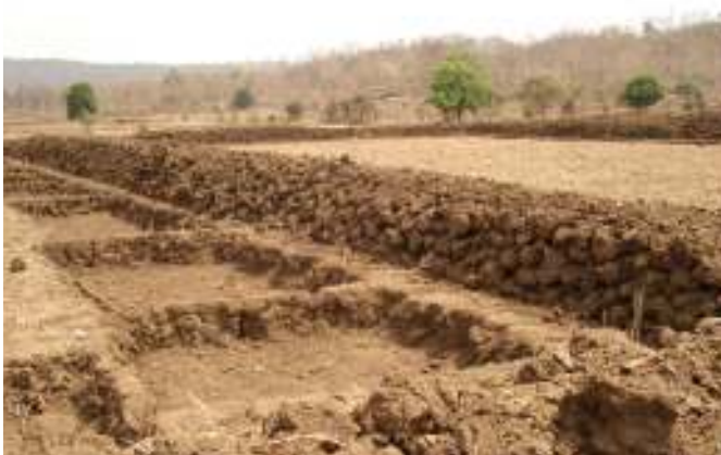
An FES facilitated farm bund at Jhulup, Mandla
