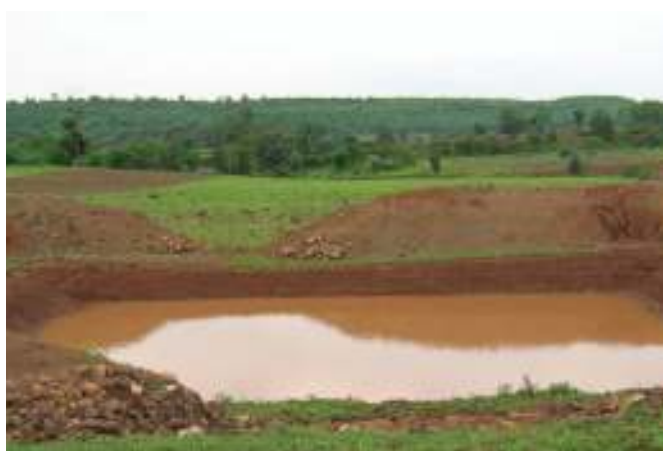
Pathadevgaon, where FES facilitated construction of a water harvesting structure
