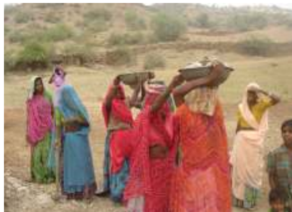
Shade at an NREGA worksite in Hallia
