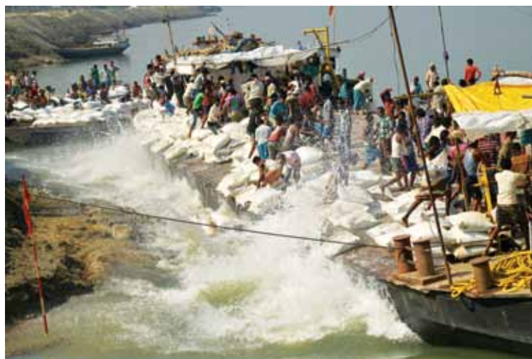
Riverbank protection with sand-filled geotextile bags in Guwahati, Assam
