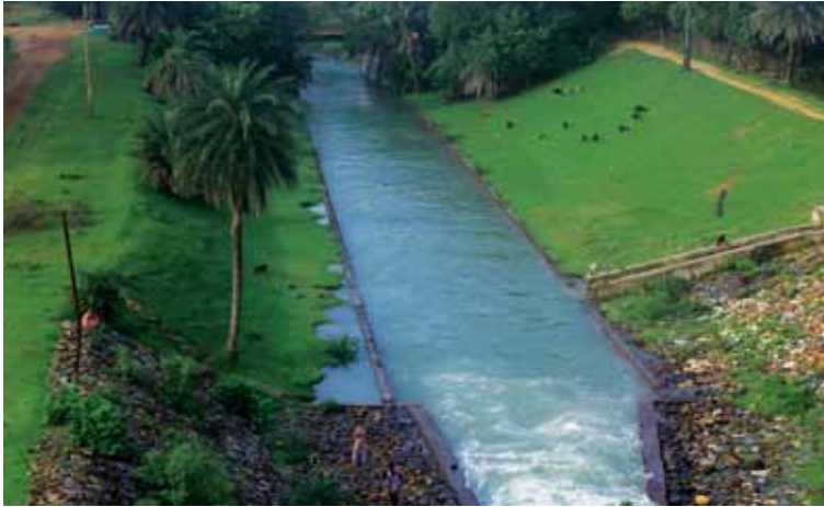
An irrigation canal upgraded under the ADB-supported OIIAWMIP, Odisha
