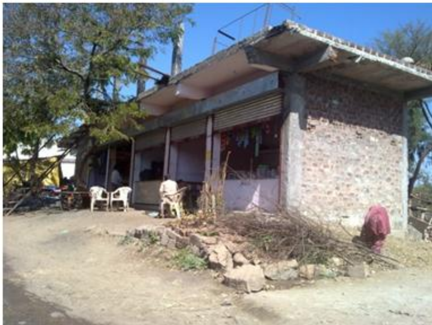
Photo 4.15: Commercial Establishments in Barkheda Salem Village
